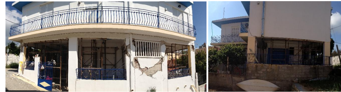
Figure 11: Comparison between the shear checks with the Nonlinear Static Procedure NSP in SeismoBuild and the actual damage sustained by the building in the 2014 Kefalonia earthquakes
