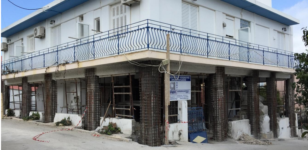
Figure 16: General view of the building during the construction of the concrete jackets
