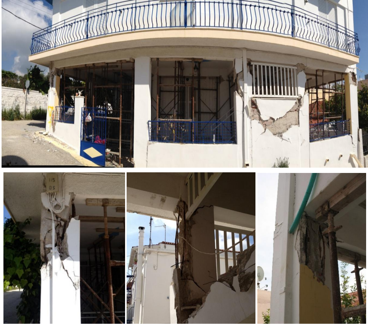
Figure 8: Damage sustained by the 2-story residential building
